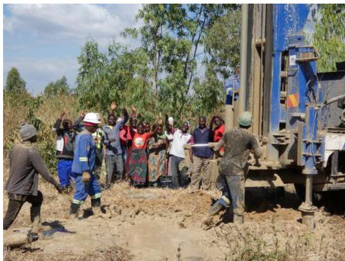
Borehole Drilling underway in Maliwata Village
